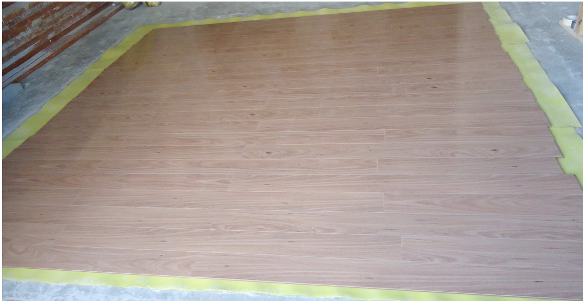
Figure 2, Laminate flooring, as installed.
